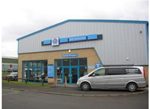
SM Autocare building on the Thornton Road Industrial Estate
