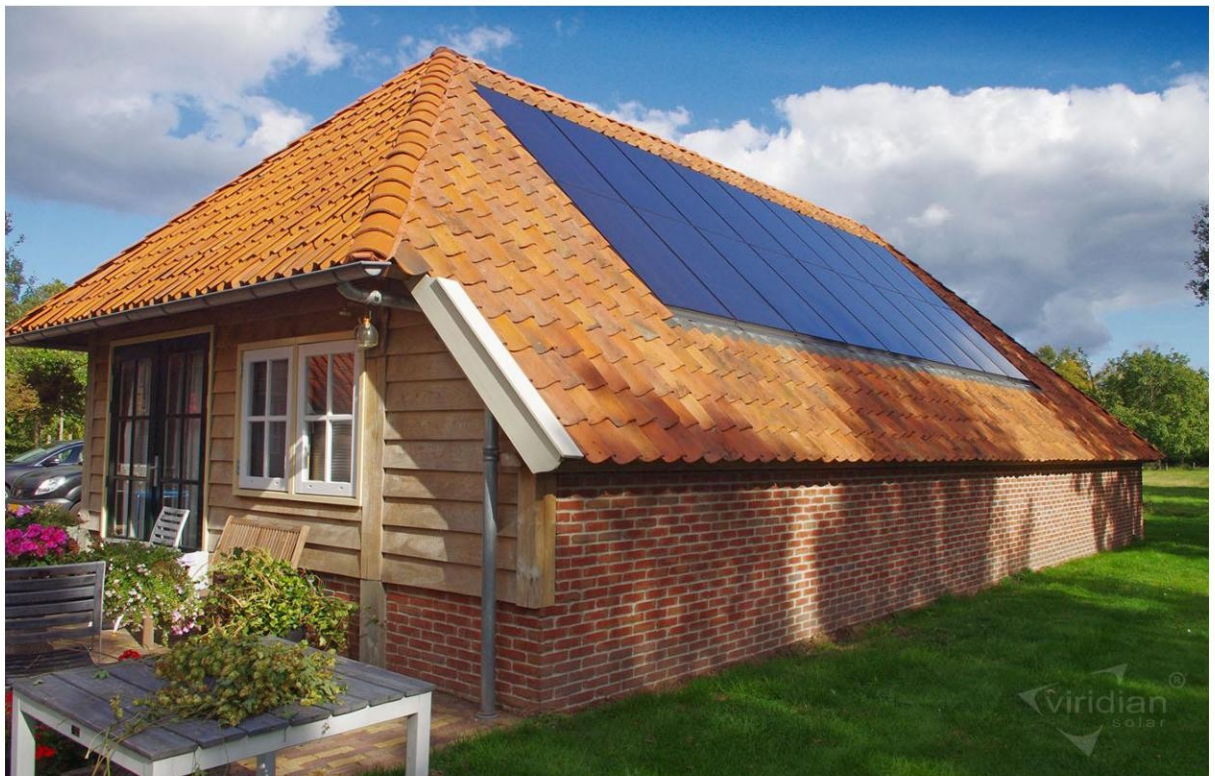
(Source: http://www.viridiansolar.co.uk/gallery-of-solar-installations.html#(grid|popup)=gallery/3151-Dakintegratie-solarpv-NL(C)ViridianSolar.jpg ; accessed 29 th April 2019)
