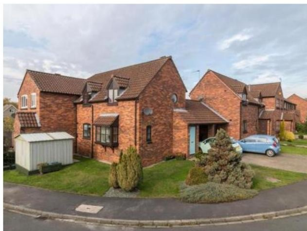
New homes on Town End Close
