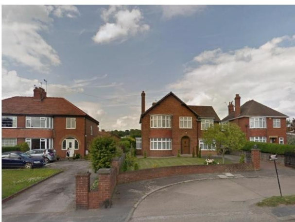
Two storey, detached homes on A170 Thornton Road
