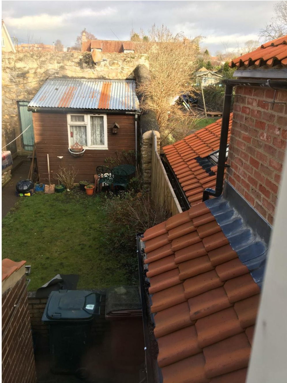
Overview of fence from the rear of 61 Eastgate
